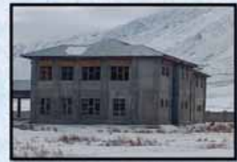
Administrative Block Work in Progress.
